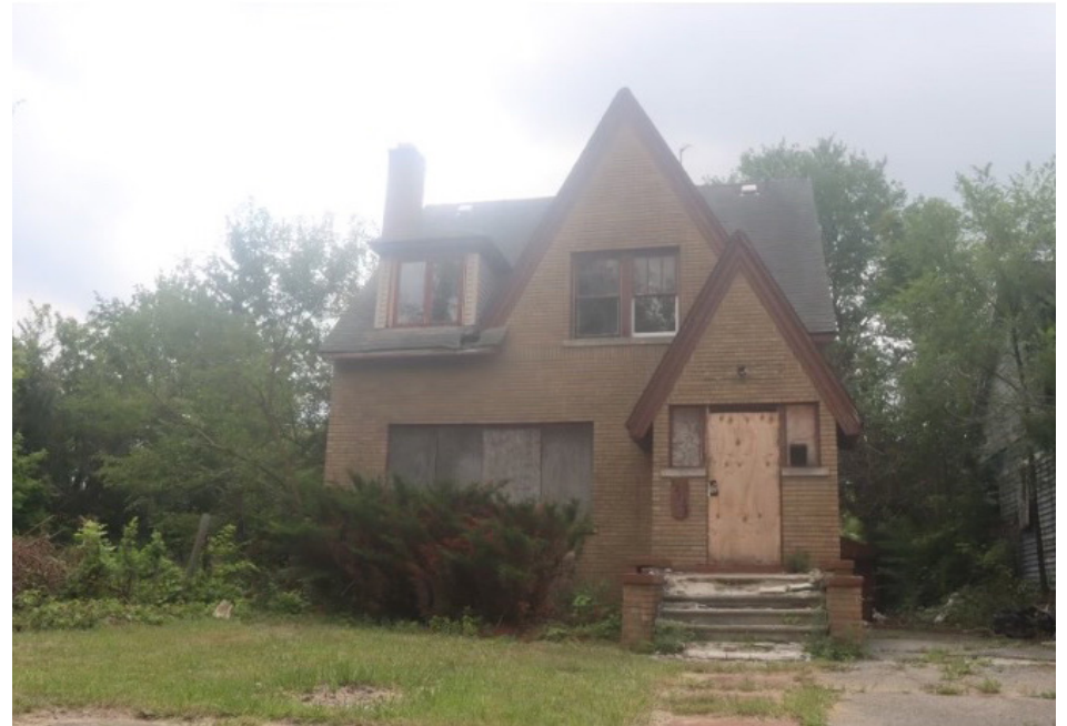
Figure 4-10: Rehabbed and Ready before
