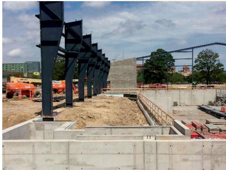
Arena under construction, midsummer of 2020: still a ways to go.
